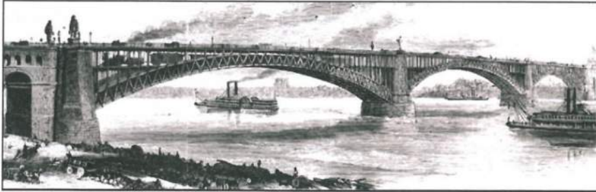
Figure 2: The St. Louis Bridge built by James Eads (Williams 1877)
