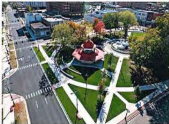
Photo: Transfer House
