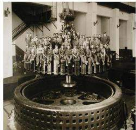
Replacing rotor, circa 1952
